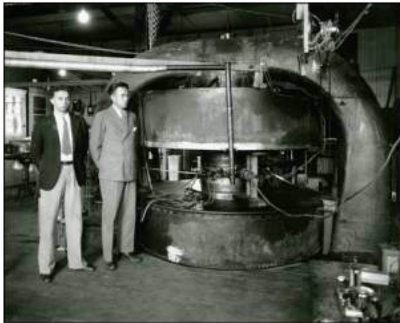
Fig. 2.9. Lawrence with 27" cyclotron in 1932 (left) and a powerful 590 MeV cyclotron built in early 1970s and still operating in Paul Scherrer Institute (Switzerland) which has a specially shape of magnets to correct for relativistic effects – particle in this cyclotron reach 78.9% of the speed of the light. The later accelerate particles from 72 MeV to 590 in 186 passes (revolutions) – each pass particles gain about 2.8 MeV.
