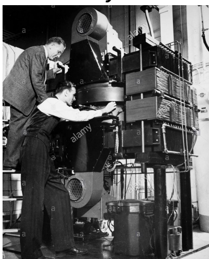
alamy stock photo 70 MeV synchrotron, GE
