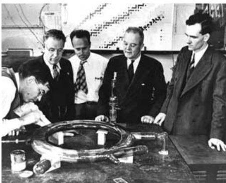
Vacuum chamber of GE synchrotron
