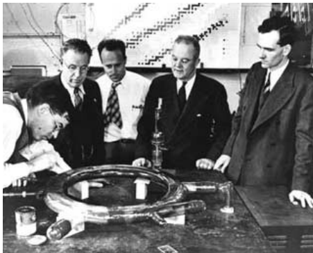
Vacuum chamber of GE synchrotron
